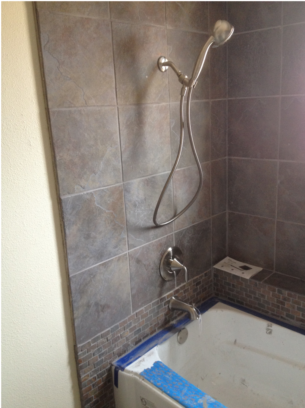
The finished job
