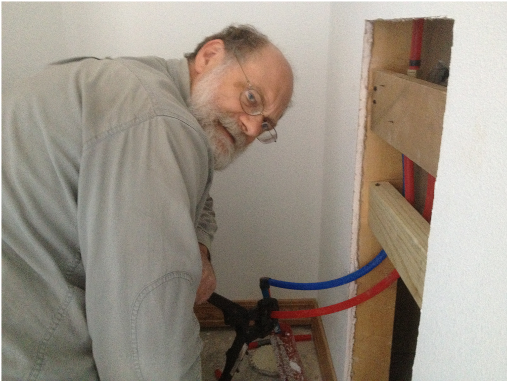
Crimping PEX plumbing connections
